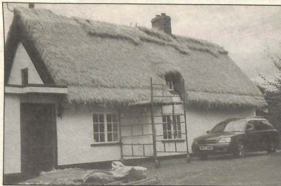
Is a thatched Roof for You? - This is Ralph and Daphne Franklin's house in Keysoe, close to Thurleigh Airfield. In the late stages of a thatching project to renew the roof over their heads, you see a rather rough rendition of the roof. And the pattern along the ridge line is the "signature" of the thatcher. The Franklins had had their name on the list for two years before the two thatchers showed up. They also had been saving more than pennies, as the bill came to more than 11,000 pounds—or as we say in the States, about $17,000 dollars. It is expected to last for 60 years or more.
